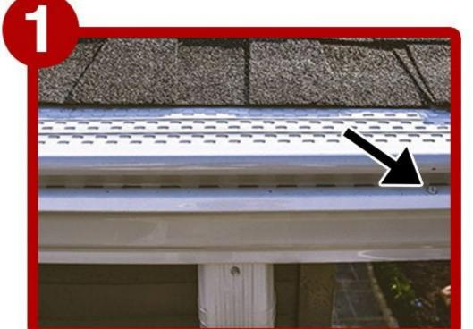
**Straight Runs:** Work left to right as viewed from the ground. Lay Waterlock Pro completely flat over existing gutters with the front edge of the panel lined up with the top front edge of the gutter and slide the back end under the first shingle.
